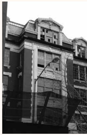
Former P.S. 64, left open to the elements for years.
