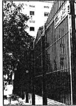
The new wrought-iron fence at Village Community School designed by Mico Sopic.
