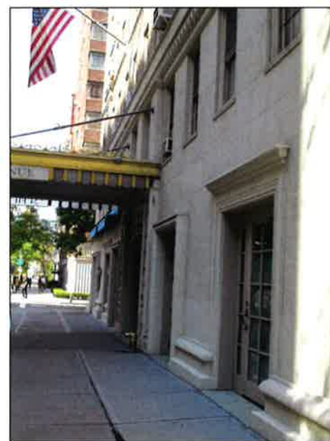
PHOTO EXISTING FACADE
