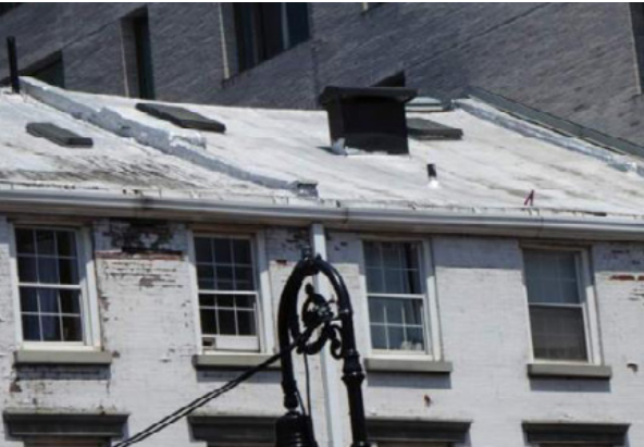
BASE FLASHING EXTENDED UP THE RISING WALL OF 14TH ST BLDG, TERMINATED WITH SURFACE-MOUNTED ALUMINUM FLASHING.
