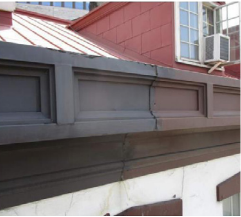
9TH AVE BLDG FORMED COPPER CORNICE OVER WOOD AND “NEW” BRICK STRUCTURE.
