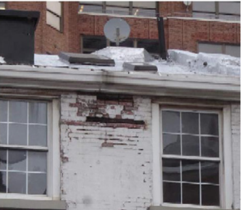
14TH ST BLDG EXPOSED DETERIORATED NAILER WOOD OF THE FASCIA BOARD IMPACTING THE STABILITY OF THE ADJACENT MASONRY.
