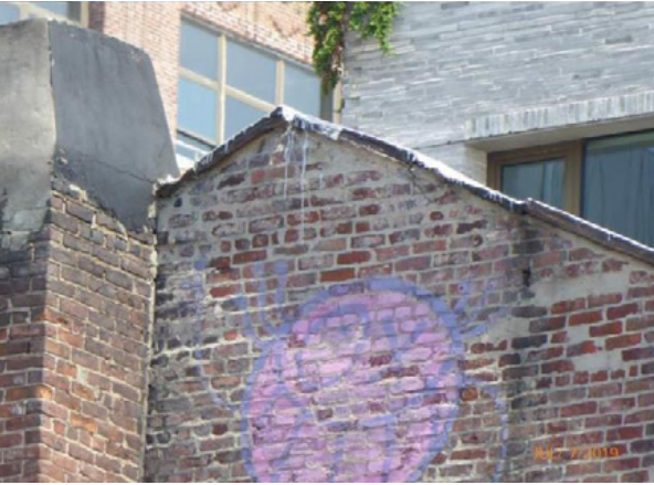
WEST FAÇADE. DELAMINATING AND SPALLED BLUESTONE COPING STONES.
