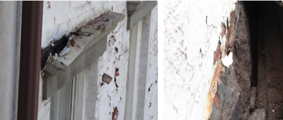
14TH ST BLDG SHEET METAL COVER OVER BROWNSTONE LINTEL
