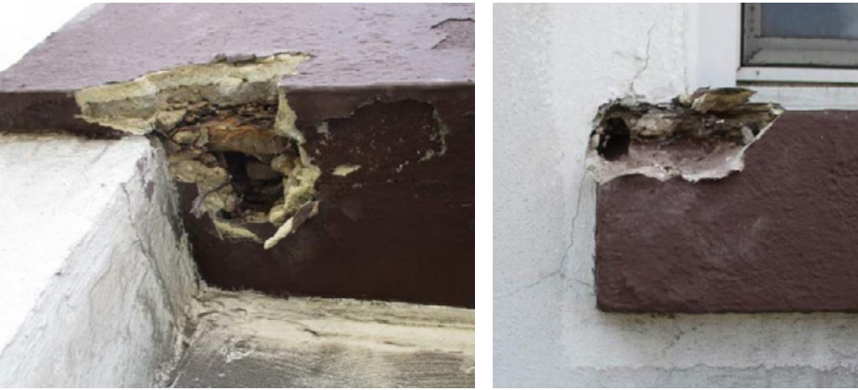
9TH AVE BLDG PROBES THROUGH REINFORCED STUCCO SYSTEM REVEALING ORIGINAL BROWNSTONE LINTELS AND SILLS
