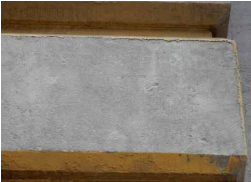
QUOIN AFTER ABRASIVE CLEANING WITH CRUSHED WALNUT SHELLS AT 40PSI
