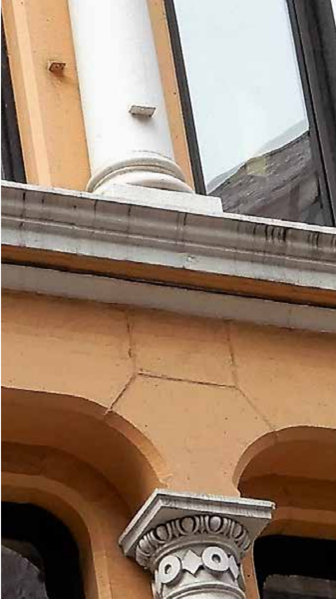
FACADE WITH EXTRANEIOUS HARDWARE, OPEN JOINTS, FLAKING PAINT
