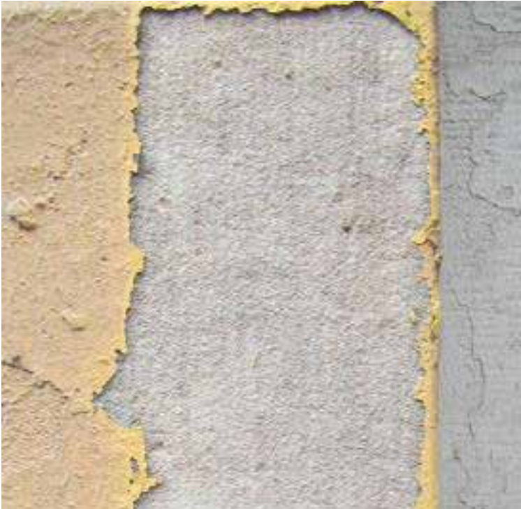
CLOSE UP OF QUOIN AFTER TEST CLEANING
