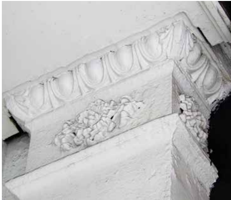
ORIGINAL CAST IRON SIDE PILASTER
