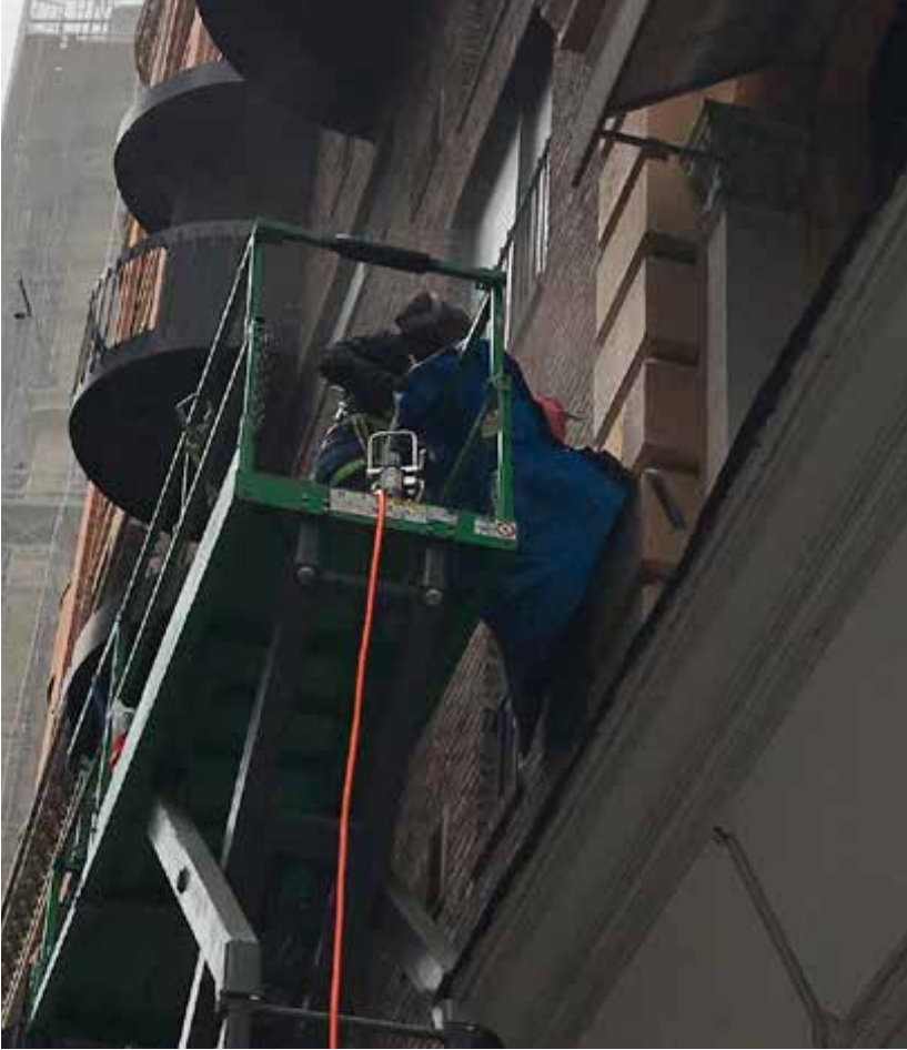
MICRO ABRASIVE TEST BEING CARRIED OUT
