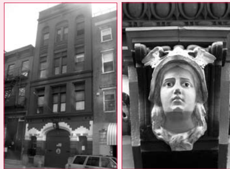
Fire Patrol House #2, 84 W. 3rd Street, with detail.
