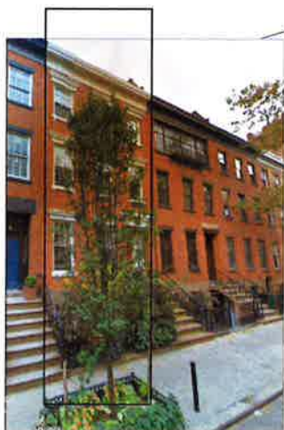
1. VIEW OF 32 PERRY STREET, LOOKING EAST.
