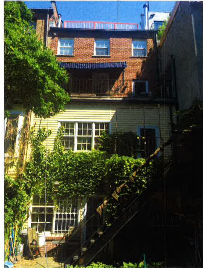
EXISTING REAR FACADE
